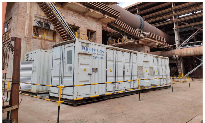
Weda Bay, Indonesia 28MWh Frequency Regulation
